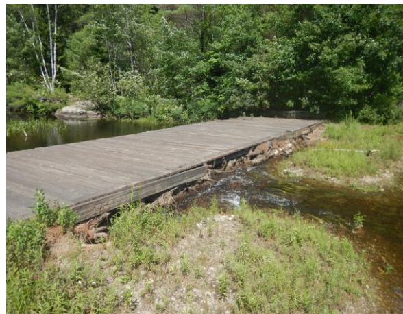
Hammond Pond Dam
